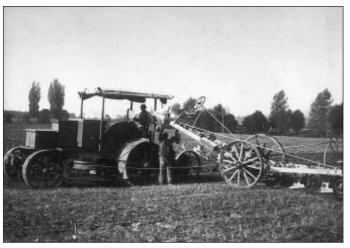
Fig. 2: Electro-plough, based on Siemens patent of 1880
