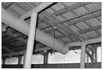
Fig. 2: Sectional view of the system for tracer gas injection with maindistributor, by-distributor and two vertical outlets
