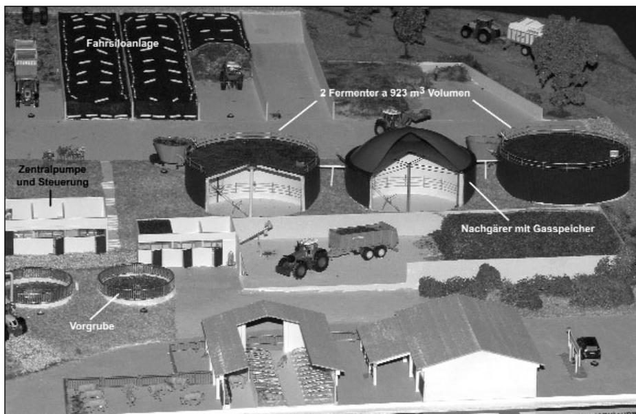
Fig. 1: Design model of the research biogas plant „Unterer Lindenhof“
