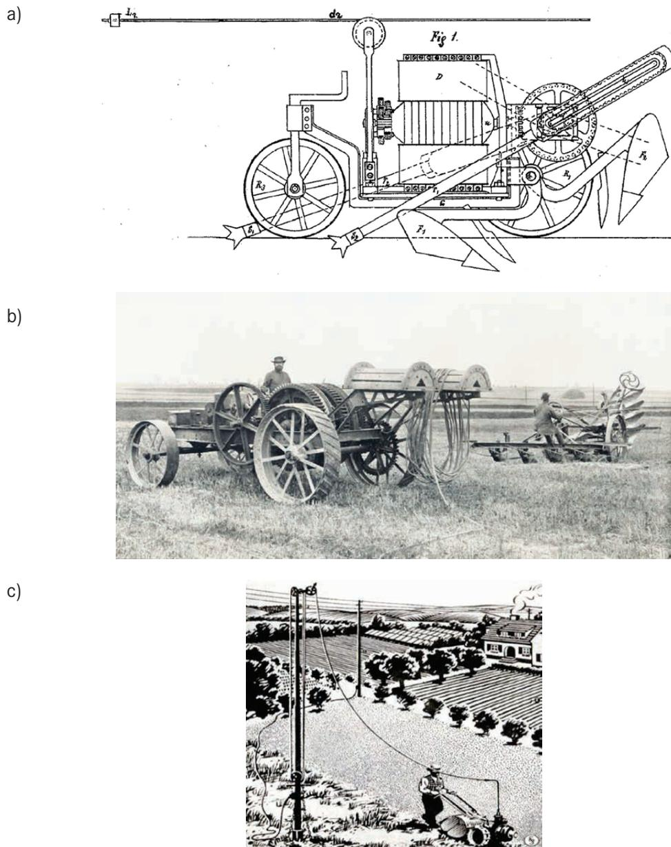
Figure 1: Early solutions for a direct electrical supply of agricultural machinery; a) Electrical plow patented by Siemens & Halske (KAISERLICHES PATENTAMT 1880) b) Cable plow equipped with an electric motor and movable anchor made by Maschinenfabrik Borsig, (BRUTSCHKE 1894) c) Solution for hand-operated machines made by Siemens & Halske (DE GRUYTER et al. 1927)
